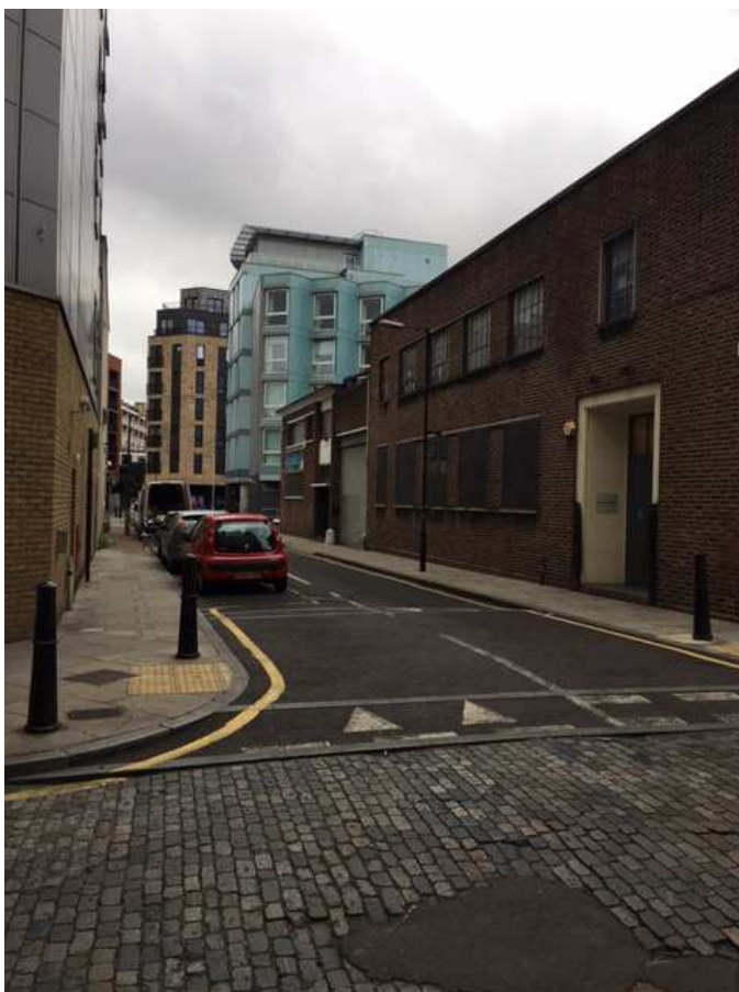
Figure 1.8: View of the existing building looking south along Herald Street
